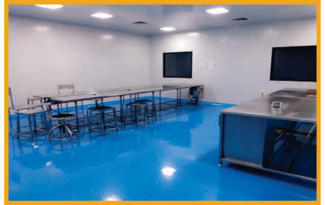
Modular Cleanroom Epoxy Coving & Flooring
